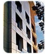
The Summerfield Suites Hotel in Charlotte, NC. The project features Dryvit's Reflect finish.
